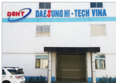
Vietnam DAESUNG HI-TECH VINA TS9 Street, Tien Son Industrial Zone, Tuong Giang Commune, Tu Son Town, Bac Ninh Province
